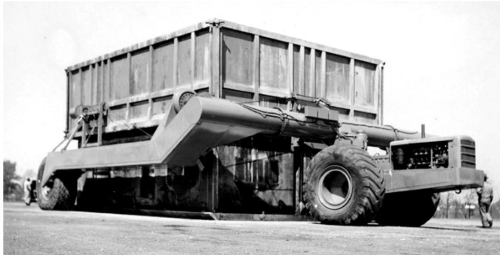
Tournalayer No. 2, Longview, Texas. Concrete house casting and laying system, 1946. The photo shows the outer form being lowered onto the inner form. Photo courtesy of the LeTourneau University Archives.
